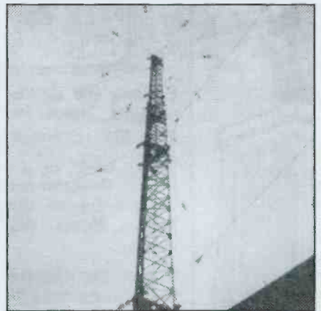
The tower at Tuckerton rose to a height of 865 feet, and supported a massive umbrella-type antenna system.
