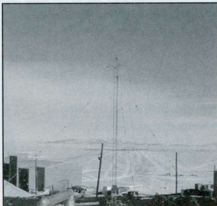
HF monopole used at McMurdo Station with ice runway operations in far background.
